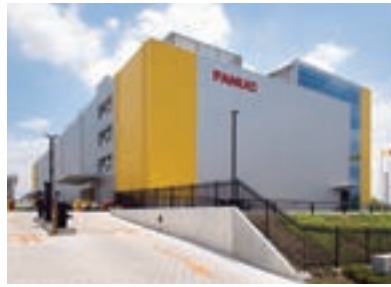
Nagoya Service Center
