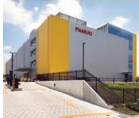
Nagoya Service Center
