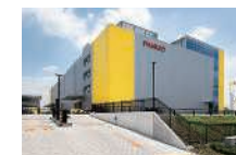
Nagoya Service Center
