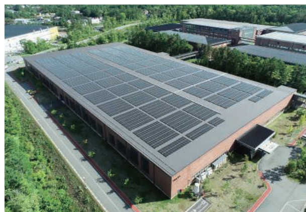
FANUC Headquarters (Reliability Evaluation Building)
